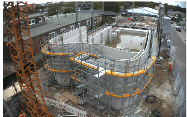
Figure 6: Heidelberg iT Management Building (Almanya) (Swinhoe, 2023).
