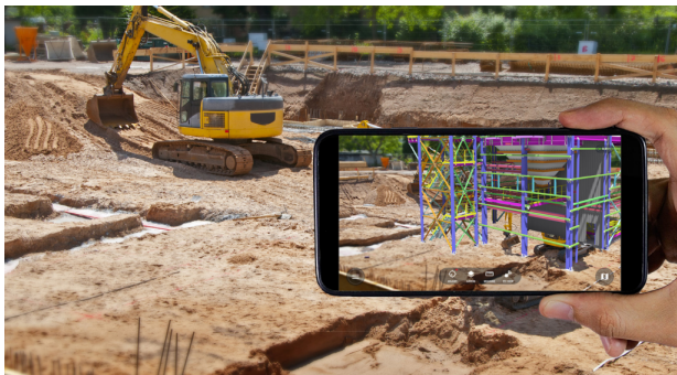
Figure 5: An example of the use of AR technology in construction (ArborXR, 2024)
